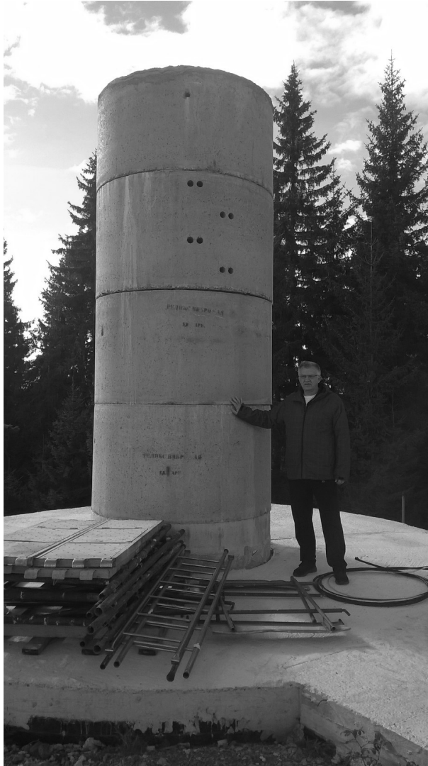
Figure 2: The concrete pillar of new 1.5 m telescope (in November 2022) at Rozhen NAO BAN (Bulgaria).
